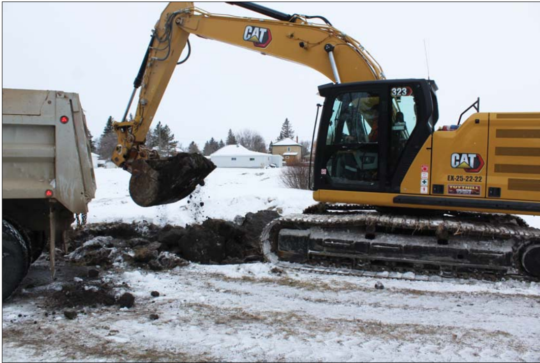
Tutthill Construction begins ground work on the new daycare in Elkhorn.
