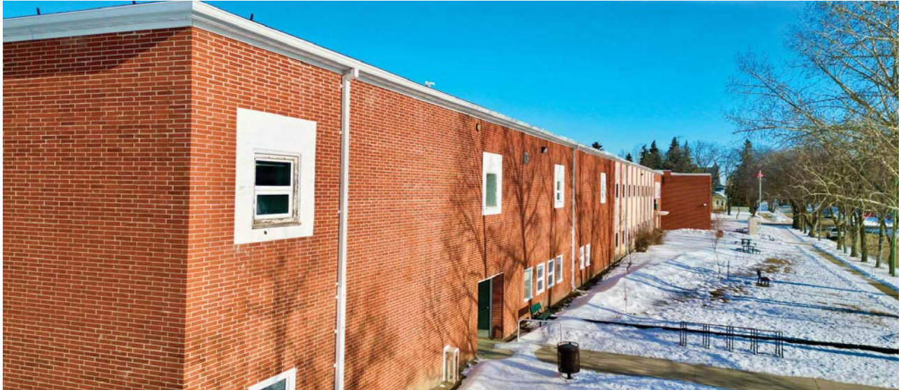
South East Cornerstone School Division has applied for up to $10 million in funding for a renovation project for McNaughton High School, above.
