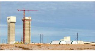
When the south shaft headframe is fully operational in March 2022, it will double the hoisting capacity at K3. Each shaft will have 36,000 tons per day hoisting capacity—for a total of 72,000 tons.
