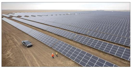
Enbridge's first solar self-power project in Canada between Lethbridge and Medicine Hat. Alberta Solar One, as it's known, supplies a portion of power to the Enbridge Mainline pipeline network, which includes the Line 3 replacement pipeline. The facility features 36,000 solar panels and has a capacity of 10.5 megawats, equivalent to meeting the energy needs to about 3,000 homes and offsetting 12.000 tonnes of carbon annually.
