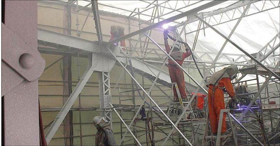
Technology has transformed the potential of painting application. Shown above are workers on Winnipeg's Redwood Bridge applying a "zinc thermal spray" - a process known as metallizing. In this metallizing process, zinc wire is melted via an electric arc and sprayed onto the steel bridge truss structure to provide corrosion protection.
