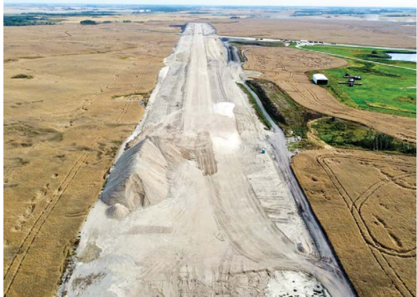
Work continues on the Moosomin airport expansion project. The new runway is oriented north-west-southeast in line with the prevailing winds.
