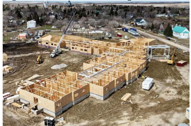
The long-term care home under construction in Grenfell.
