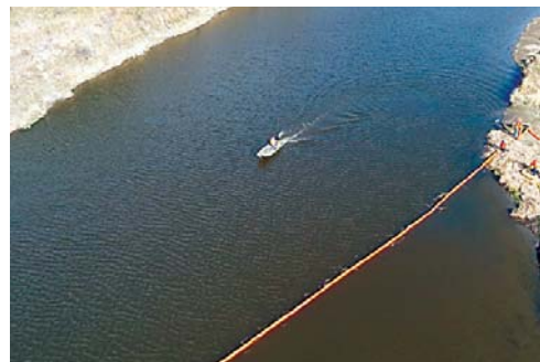
Above: Boom deployment across the Souris River, captured by a drone.
