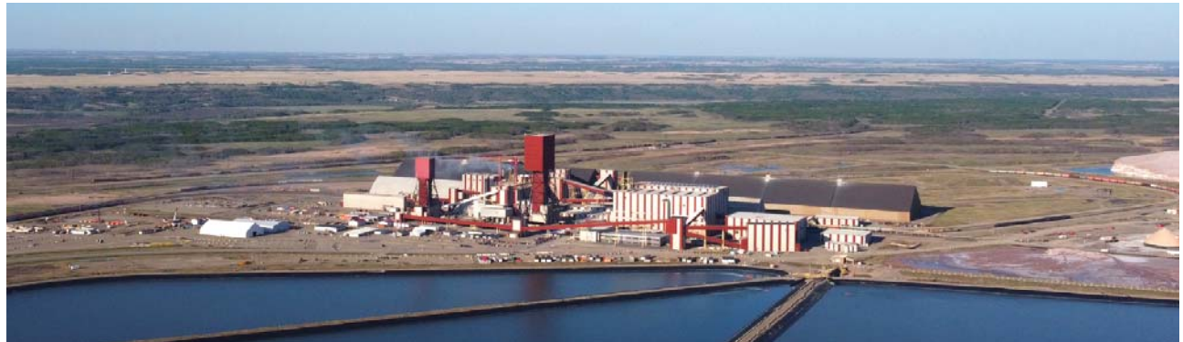
The Nutrien potash mine at Rocanville. Work is underway on a multi-year refurbishment of the original mill, replacement of underground raw ore bins, and the addition of a power generating plant. The contractor workforce will peak at between 500 and 1,000 for the next three years.
