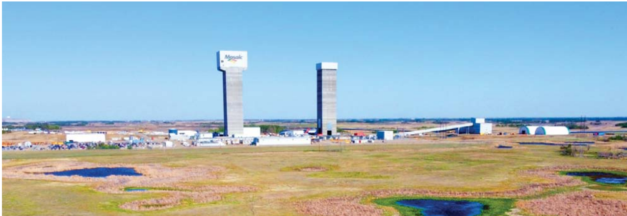
Mosaic's K3 potash mine at Esterhazy in a recent shot by Kevin Weedmark. K3 should be up to full production in less than a year. K1 and K2 were to keep operating until production ramped up at K3, but increased brine flow led to the closure of both the K1 and K2 shafts.
