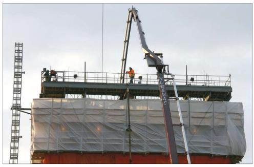
Workers on the top deck above the slipform as concrete is pumped into the form. Workers up top place rebar and finish the concrete as the slipform rises.
