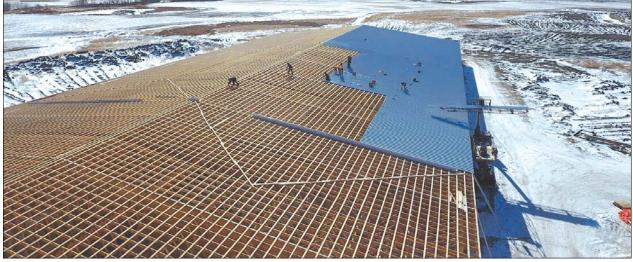
Work on the roof of the massive new hog finishing barn at the Plainview Colony. The massive building measures 172 feet by 710 feet. It will ship out 700 hogs a week to the Maple Leaf plant at Brandon. See inside for more photos.
